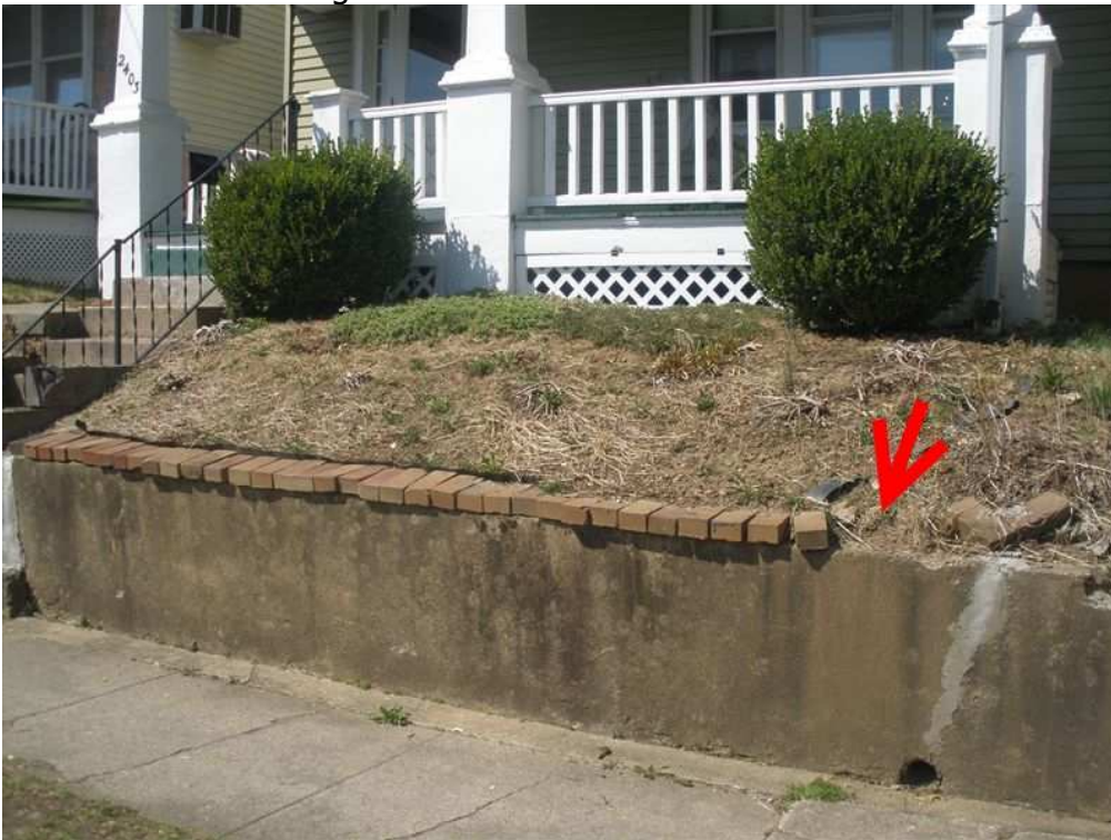
Photo #3 the retaining wall
