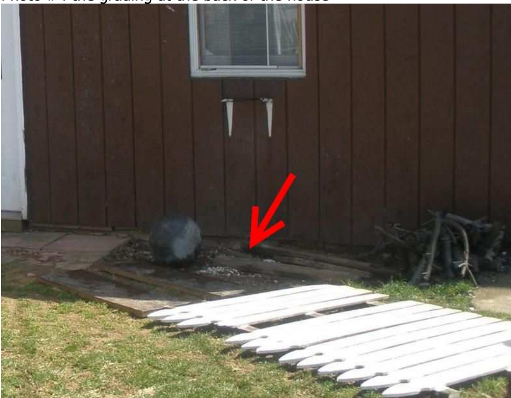
Photo #4 the grading at the back of the house
