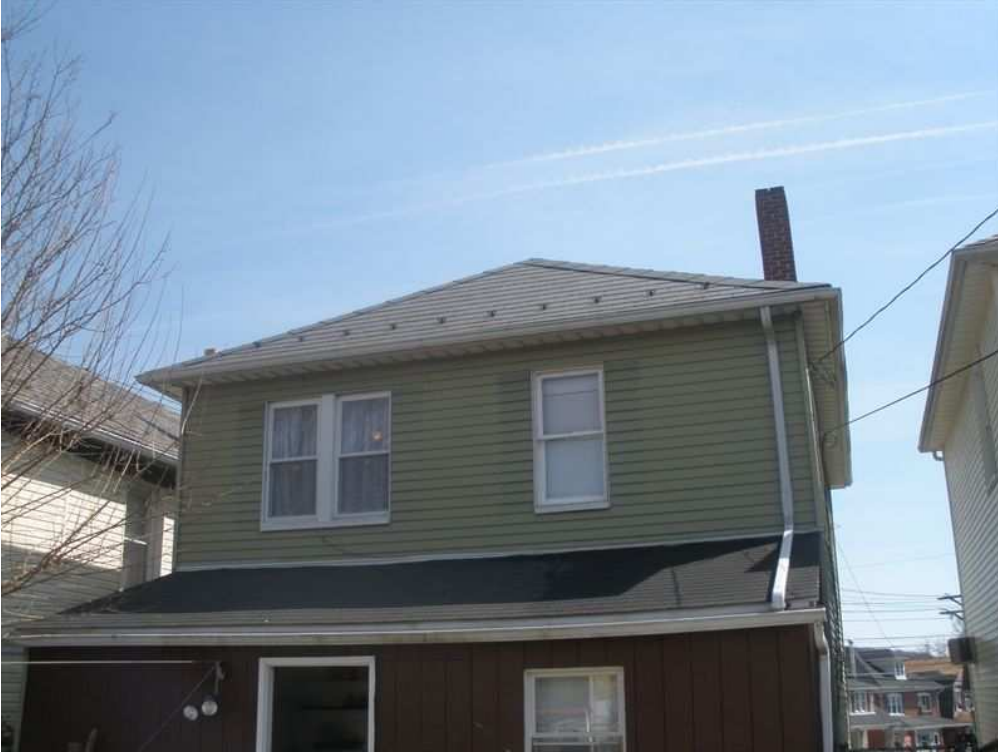
Photo #9 Roof style
