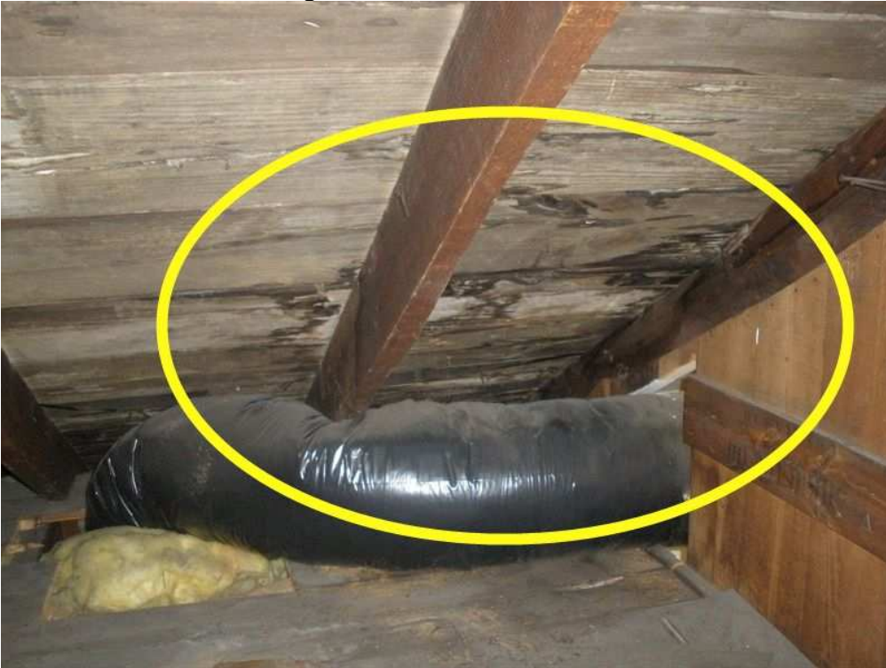
Photo #20 attic sheathing
