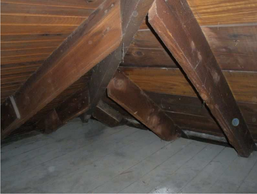
Photo #19 roof frame
